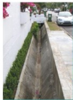
Open roadside drain
